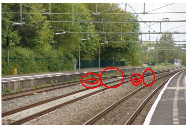
Figure 154: The red circles indicate two dwarf signals that should be two normal signals with progressive speed signs on paper. Furthermore, two static speed signs are missing and the signal numbers are incorrect.
