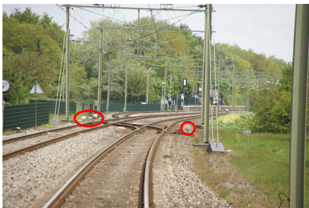
Figure 159: Proves that three switches are characterized by a wrong number.
