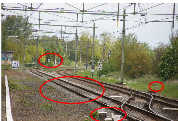
Figure 158: The standard static speed sign 8 in the back should be a triangle facing downwards with an 8. In addition, all three switch numbers are incorrect. Again the static speed sign 10 towards Bv on the left track misses as well.
