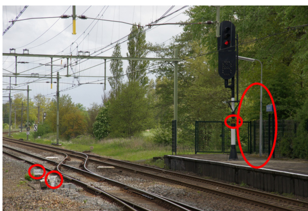
Figure 157: This figure also finds that the switch numbers are incorrect and the signal number at track 1 is incorrect.
