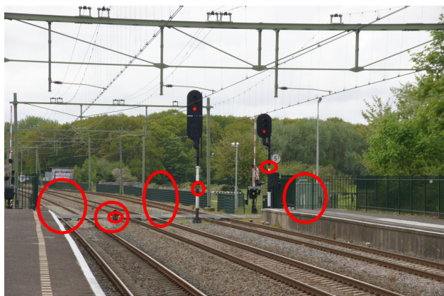
Figure 149: The red circles mark wrong signal numbers, missing static speed signs and a dwarf signal which should actually be a normal signal.
